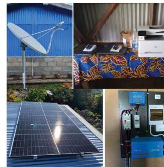
Installation at Melken Community, Malekula
